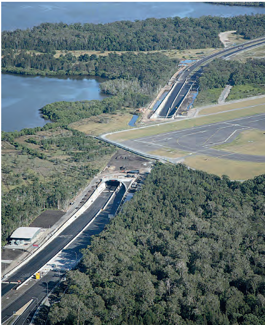
The Tugun Bypass Tunnel constructed under the extension of the main runway of the Gold Coast Airport.
